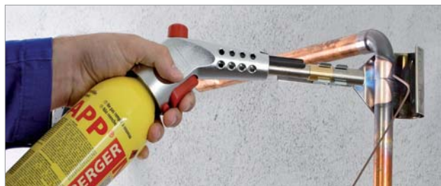
Brazing in gas installation
