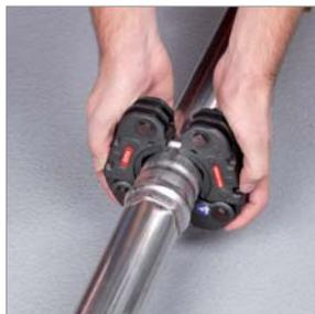
Gripping the pressing collar with intermediate jaws
