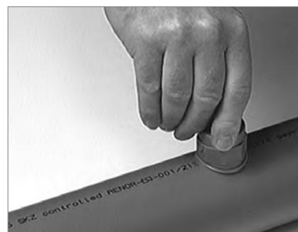
After a cooling time of 10 minutes the fused joint can fully work under pressure.
